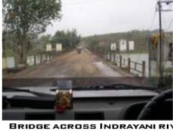
BRIDGE ACROSS INDRAYANI RIVER
